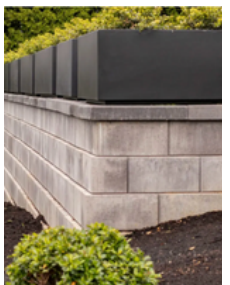
MURUTA BY: WESTERN INTERLOCK
