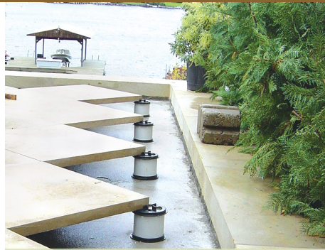
Hydrapressed slabs over a concrete patio
